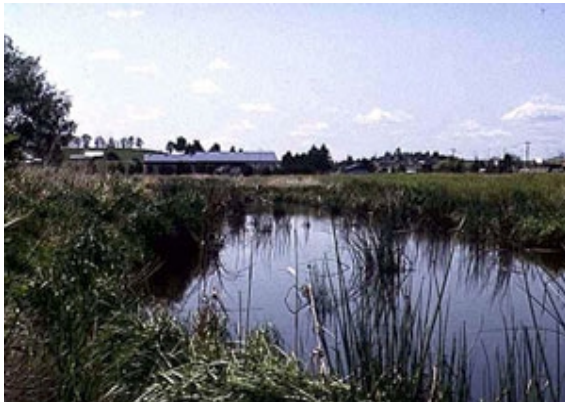
Moscow Wastewater Treatment Plant
