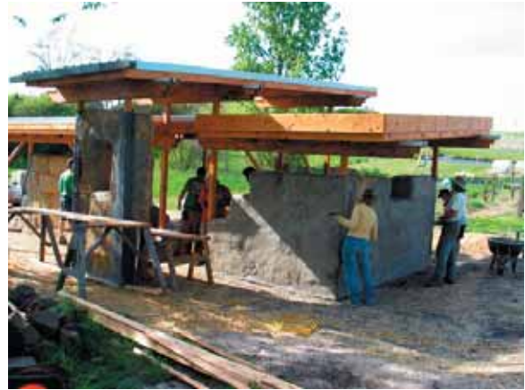
Volunteers and PCEI staff work with Kurt Rathmann on the first coat of stucco. Photo: Sara Lynd
