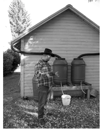
Moscow resident, Jason Mills demonstrates how his rain water collection system works on the back of his shed. Jason uses his water to grow corn, peppers and tomatoes in front of his home on A street. Jason built the system mostly with recycled materials and collects 165 gallons at a time. Photo: www.pcei.org
