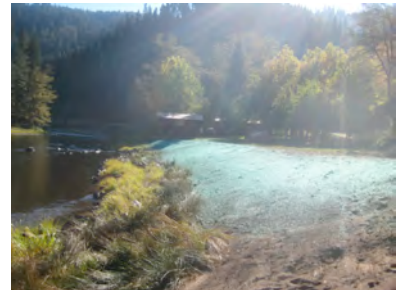
Post Excavation September 2010
