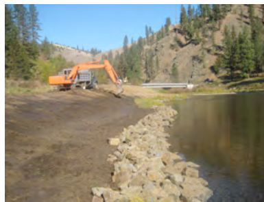
During Excavation September 2010
