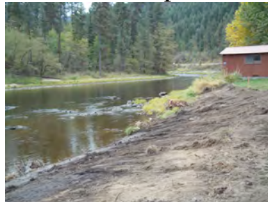
During Excavation September 2010
