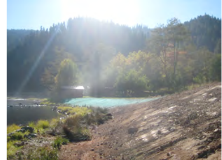
Kirtner, October 2010: Sedge mats were installed to help strengthen the toe and stabilize the banks.
