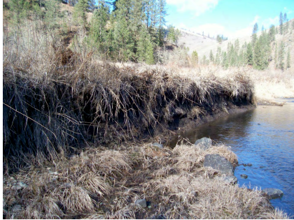
Kirtner, October 2005: Eroding bank with be stabilized during restoration efforts in order to reduce sediment loading to the South Fork Clearwater River.
