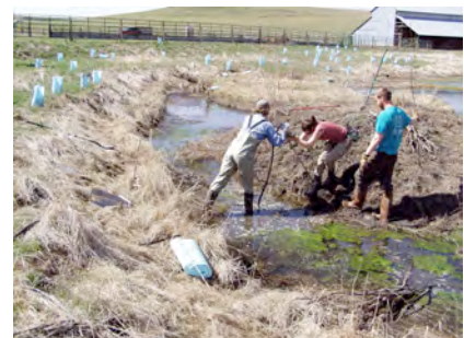
April 2010: PCEI 2010 AmeriCorps members plant willow poles in the wetland near Luke's Gulch road using a stinger and teamwork.
