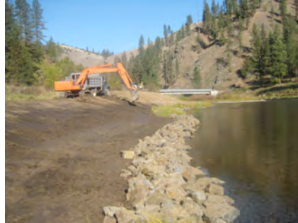
Kirtner, October 2010: Banks stabilized with 3:1 slopes and a rock toe.
