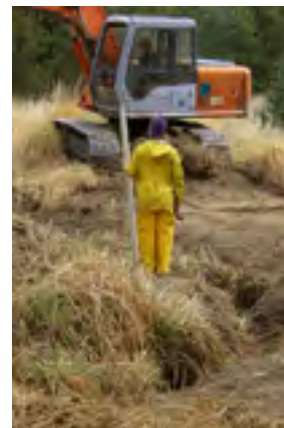
October 2007: Sara Cucksey, PCEI Project Manager directs construction crew.
