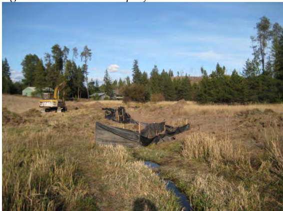
October 2008: The banks of the Reynolds' property Flannigan Creek are resloped to minimize erosion. The black fencing helps to minimize disturbance to the creek from rollback and runoff in case of a rain event.
