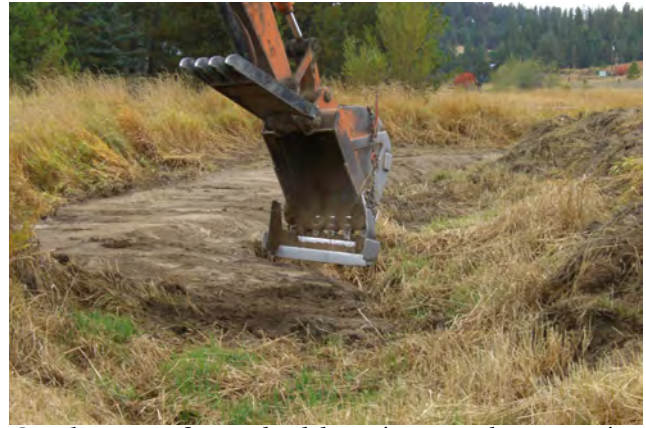
October 2007: Stream bank berm is removed reconnecting floodplain to the creek.
