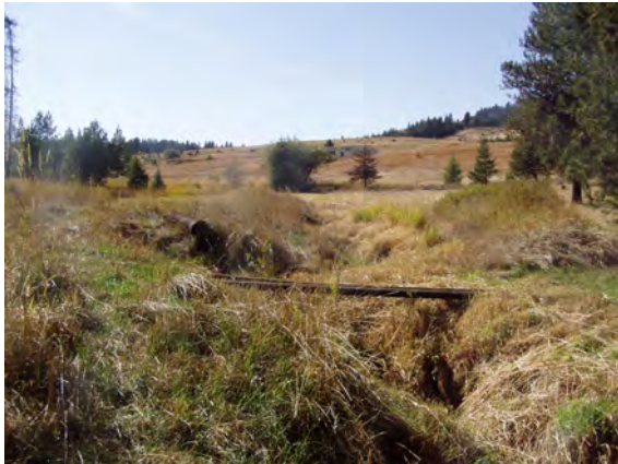
September 2007: Photo point 3 upstream. Prior to restoration. Steep, unstable and actively undercutting banks throughout the restoration project.
